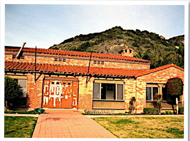
HISTORIC SHELL CLUBHOUSE
